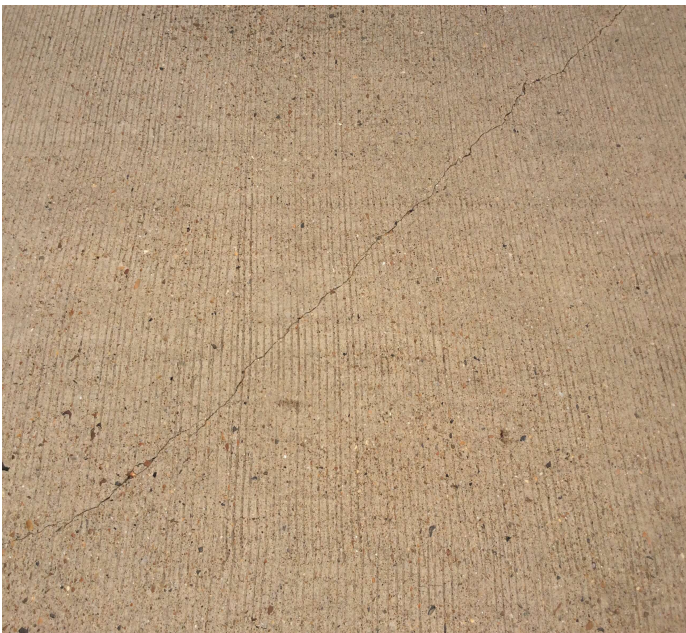
PHOTO 1 Description Deck cracks
