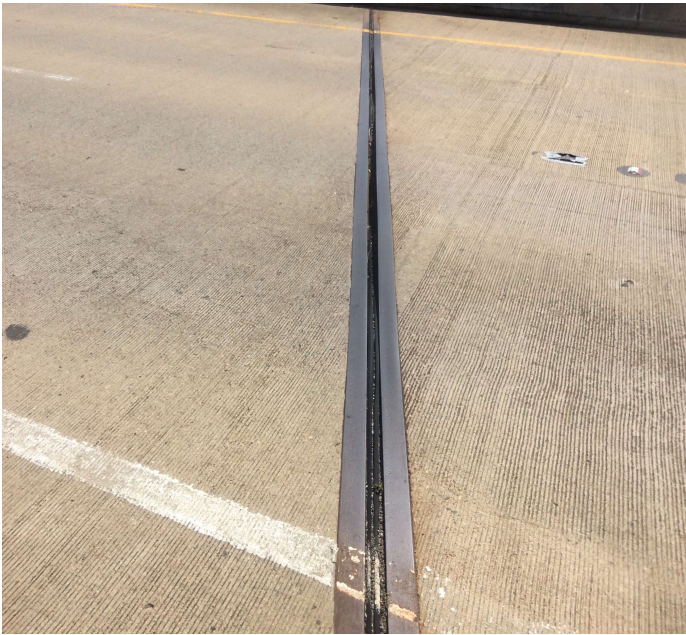
PHOTO 1 Description 20' of joint seal in eastbound lane at bent 3 has fallen out.
